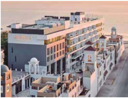
ARABELLA HOTEL, KUWAIT Al Vida, Kuwait Architect Agency: SQC International Fabricator: Al Khalid Aluminium
