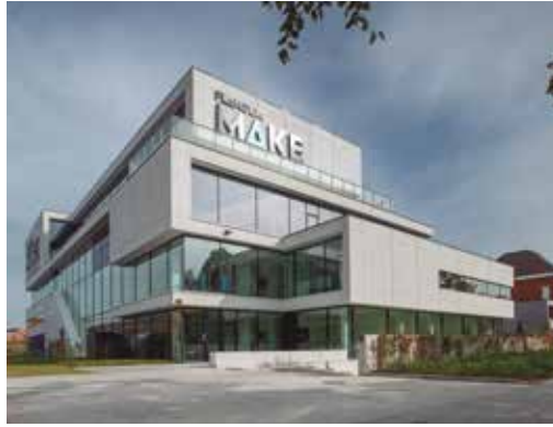
FLANDERS MAKE Kortrijk, Belgium Architect Agency: Jaspers-Eyers Architects Fabricator: Durv
