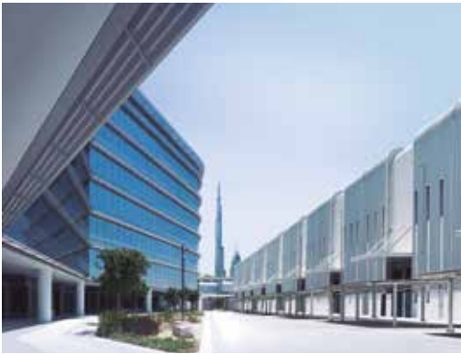
DUBAI COMMERCITY Dubai, United Arab Emirates Architect Agency: P&T Group Fabricator: Al Barary Aluminium and Glass L.L.C.
