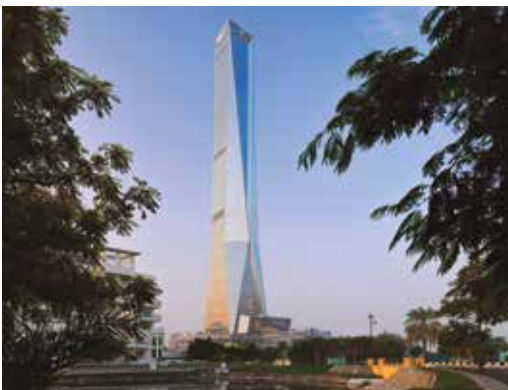
DUBAI UPTOWN TOWER Dubai, United Arab Emirates Architect Agencies: AS+GG & Woods Bagot Fabricator: Besix
