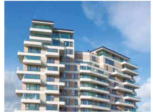
THE ONE BLANKENBERGE Blankenberge, Belgium Architect Agency: A1AR Fabricator: Inghelbrecht Construct
