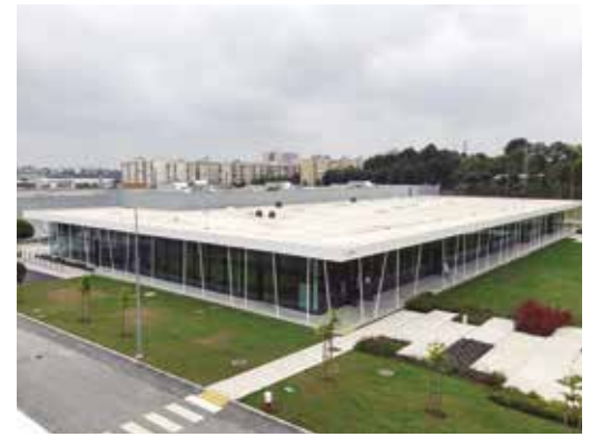
BOSCH BRAGA INDUSTRIAL COMPLEX CANTEEN Braga, Portugal Architect Agency: Rodapé Arquitectos Fabricator: Trivglass
