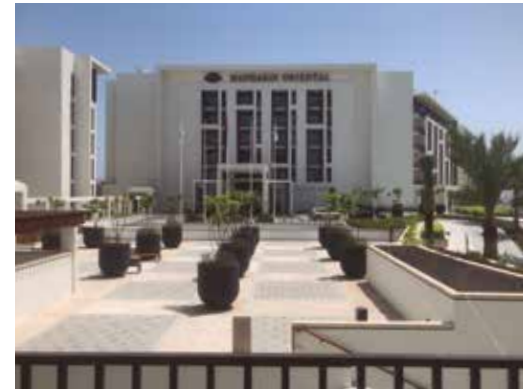
MANDARIN ORIENTAL HOTEL Muscat, Oman Architect Agency: SSH Fabricator: Airmech Oman LLC
