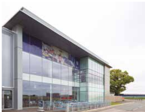
SILVERSTONE EXPERIENCE Northamptonshire, United Kingdom Architect Agency: Cube Design Fabricator: Quality Glass
